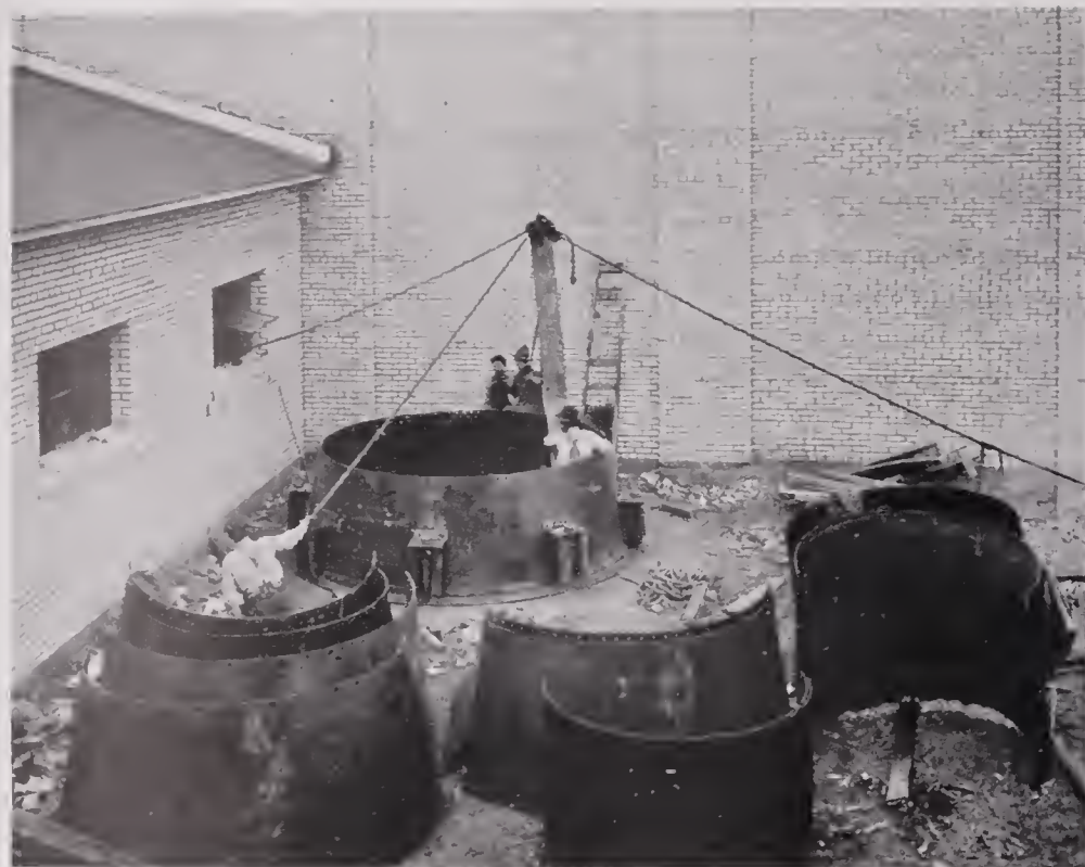
ERECTING FORGE POWER PLANT STACK
